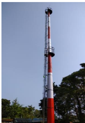
Spun Concrete Tower 15 Mtrs – 14 Nos. 30 Mtrs – 27 Nos.
