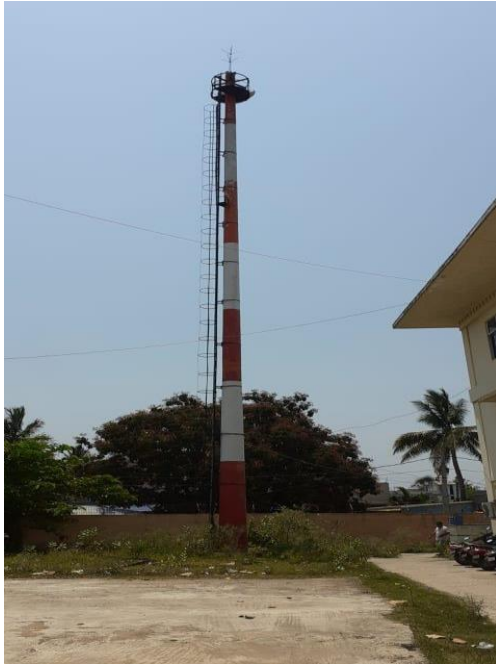
Spun Concrete Tower
