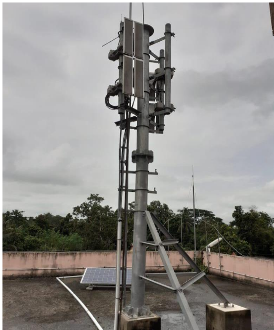
Roof Top Tower
