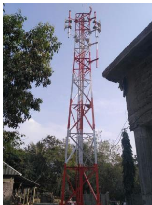
Angular Tower 15 Mtrs – 33 Nos. 30 Mtrs – 29 Nos.
