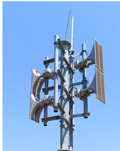
Siren installed at tower top
